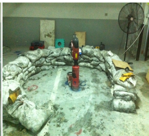
Figure 3 – Diamond Core Drilling Set Up
