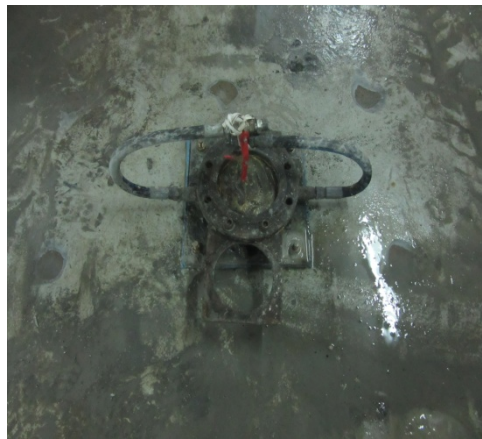
Figure 4 – Flange Head Plate & Gate Valve
